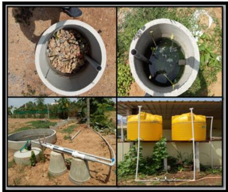
Fig. 2. Field established grey water treatment unit
