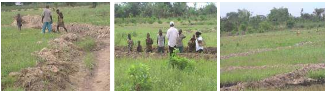
Fig. 3. Construction of interceptive canals and bund making for sawah field development
