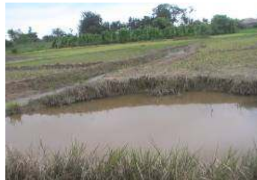
Fig. 2. Constructed canal from the spring source and the artificial pond for supplemental irrigation
