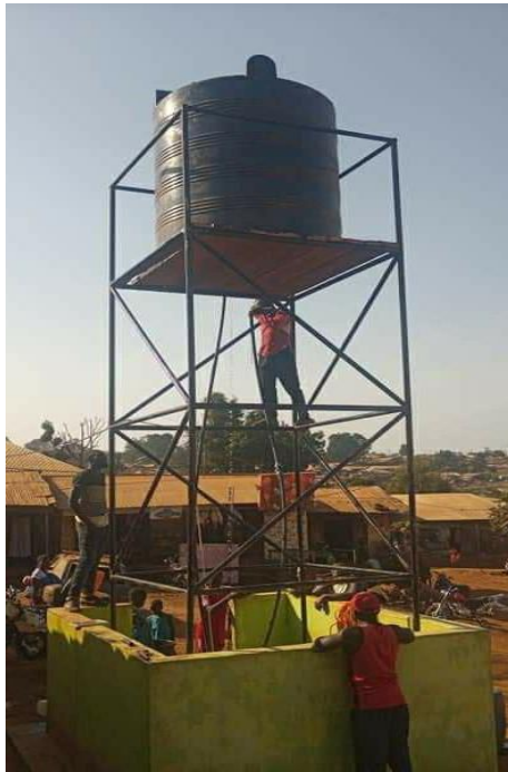
Fig. 5. Village borehole in a market square
